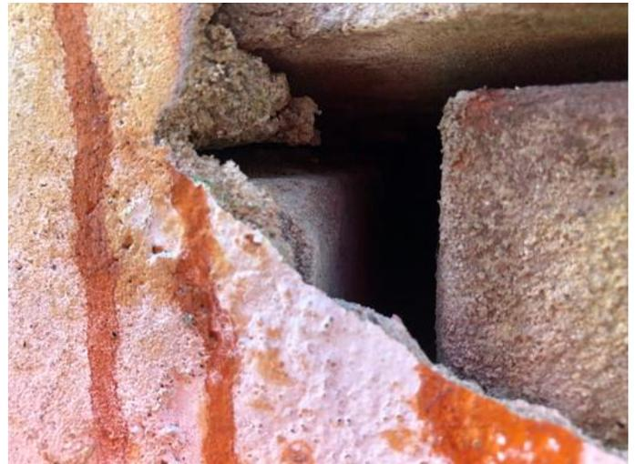
Deep holes found within masonry where water is most likely leaking into.
