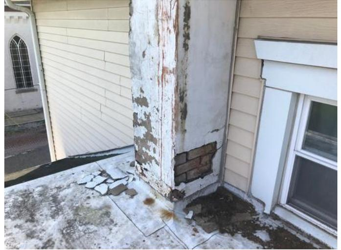
Concrete wash on chimney's exterior is chipping away in large sections exposing interior brick.
