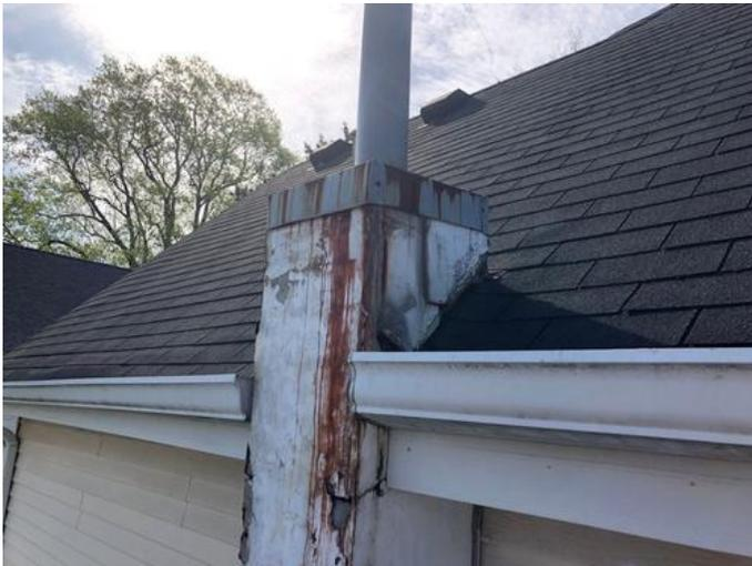
Chimney is not flashed properly at either roofline.
