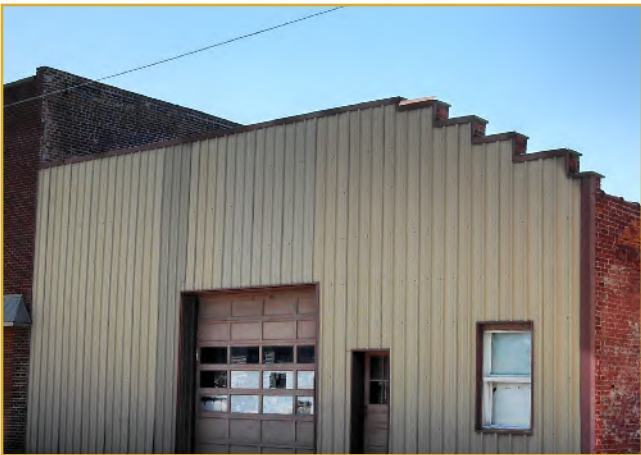
Above: Parapet wall example
